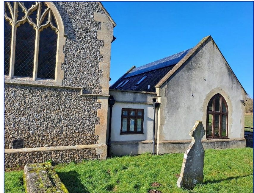
Principal and prominent pitches should be kept free from Solar Panels, to minimise visual impact, or placed on extensions or buildings of less significance
